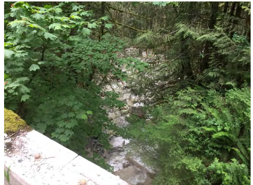
Looking downstream from deck
