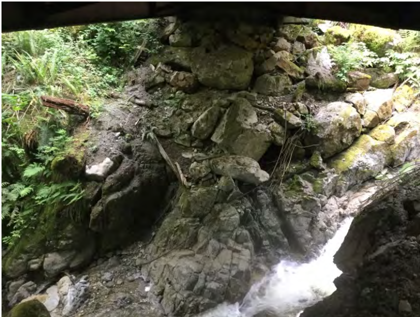
Right Bank Abutment when facing downstream
