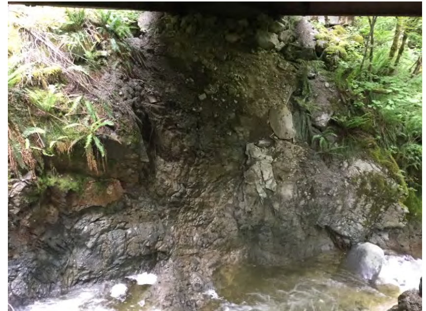
Left Bank Abutment when facing downstream
